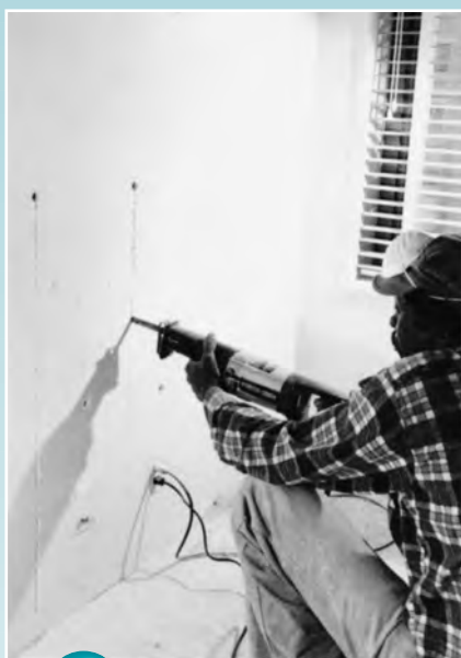
7 Cutting wall openings
