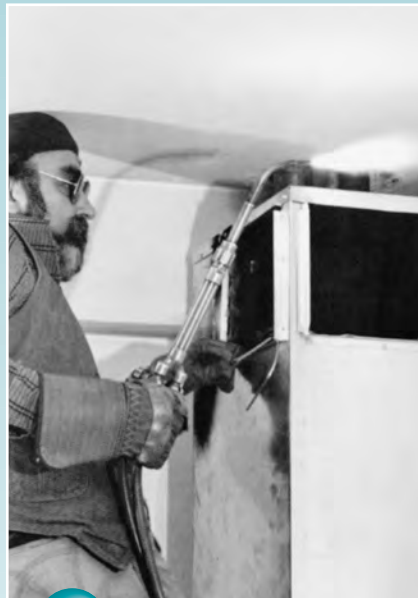
Joining risers to unit above
