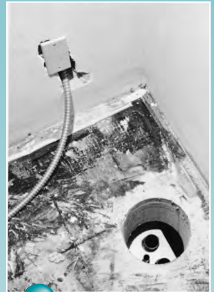
Top of unit below visible in core hole
