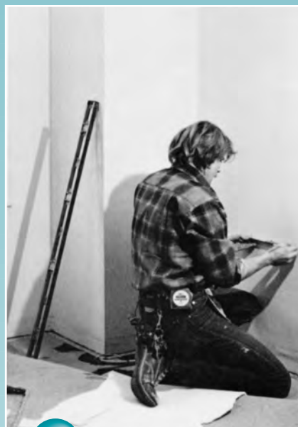
2 Measuring and marking grille width
