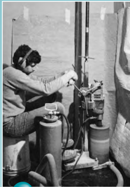
Core-drilling floor
