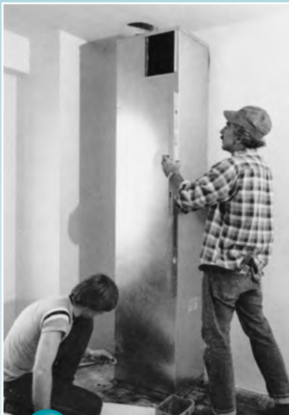
Levelling fan-coil unit
