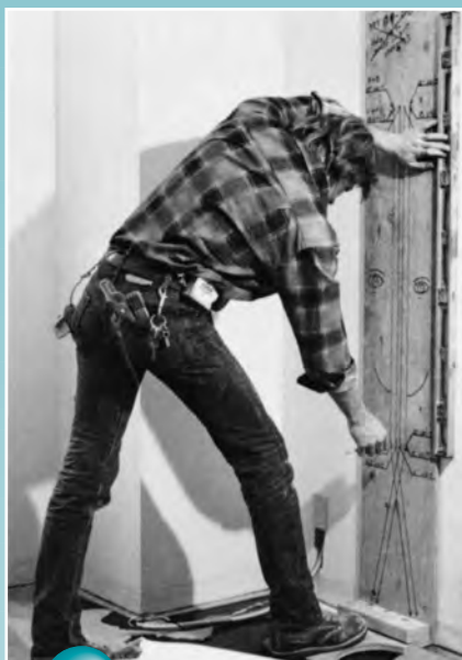
1 Template locates center of grille openings
