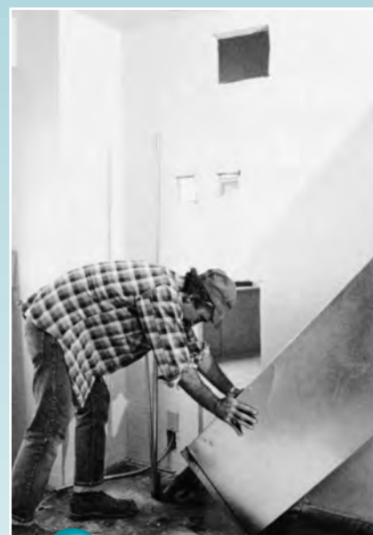
9 Tipping unit into place
