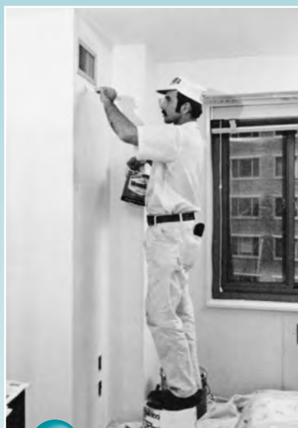
17 A final coat of paint
