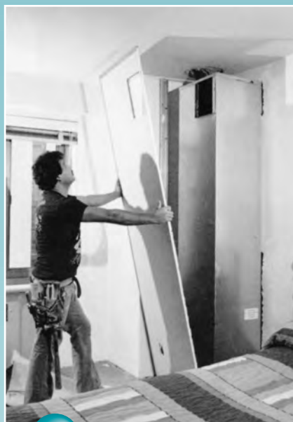
14 Applying "drywall" gypsum board
