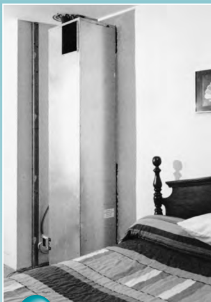
13 Unit ready for gypsum board
